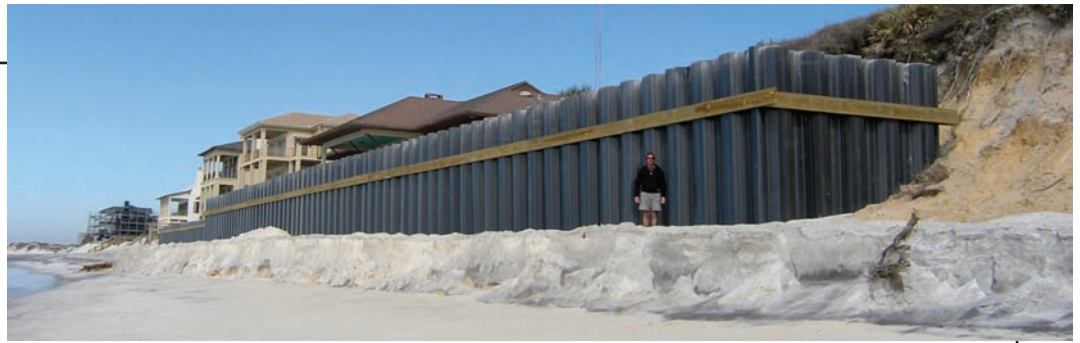
Sea wall west of Blue Mountain Beach in Walton County Florida.
